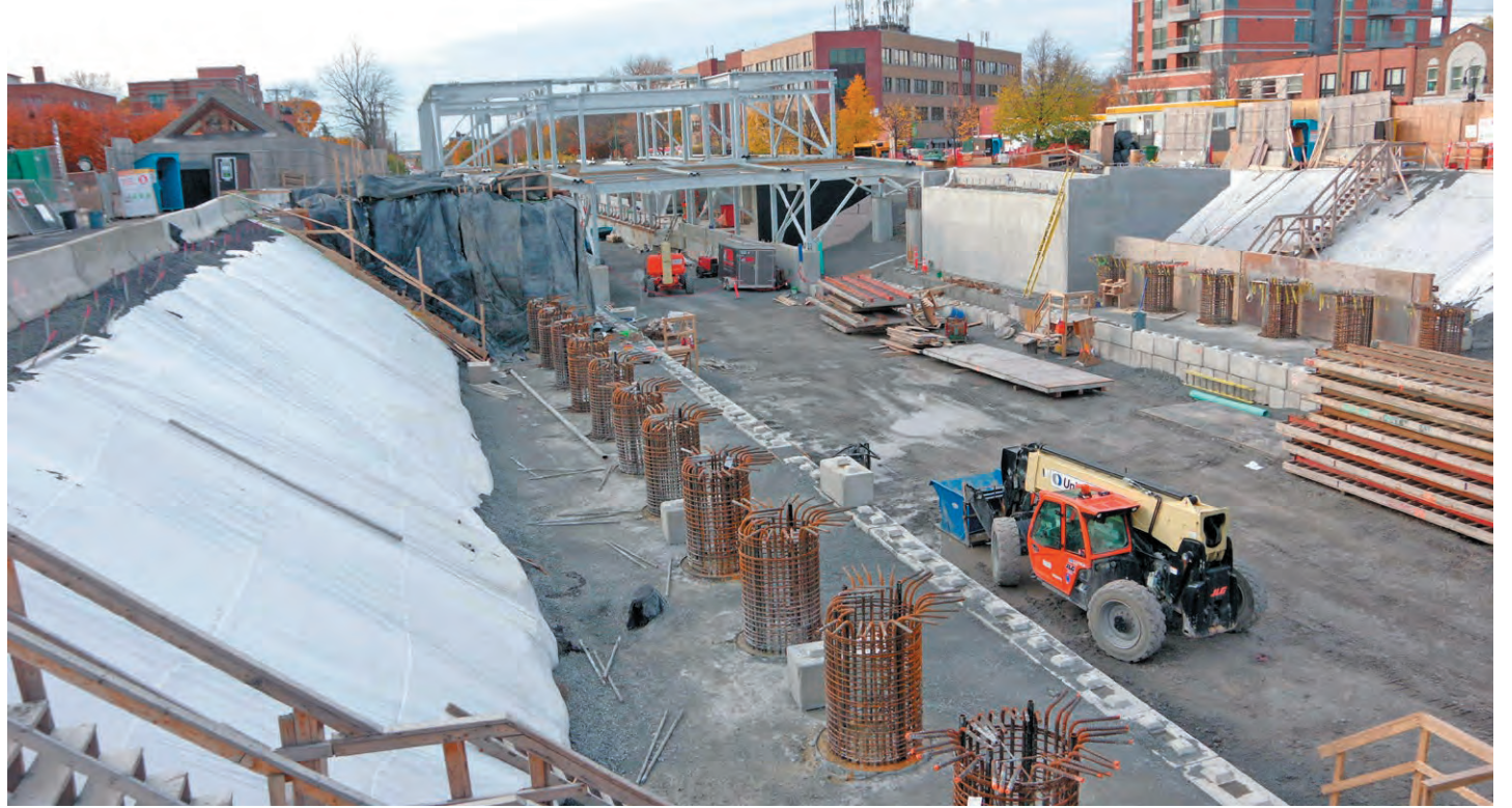
CDPQ Infra's rapid transit REM line, now under construction through the heart of TMR, is the focus of The Train that Tricked Us , which takes issue with the developer's methods.
