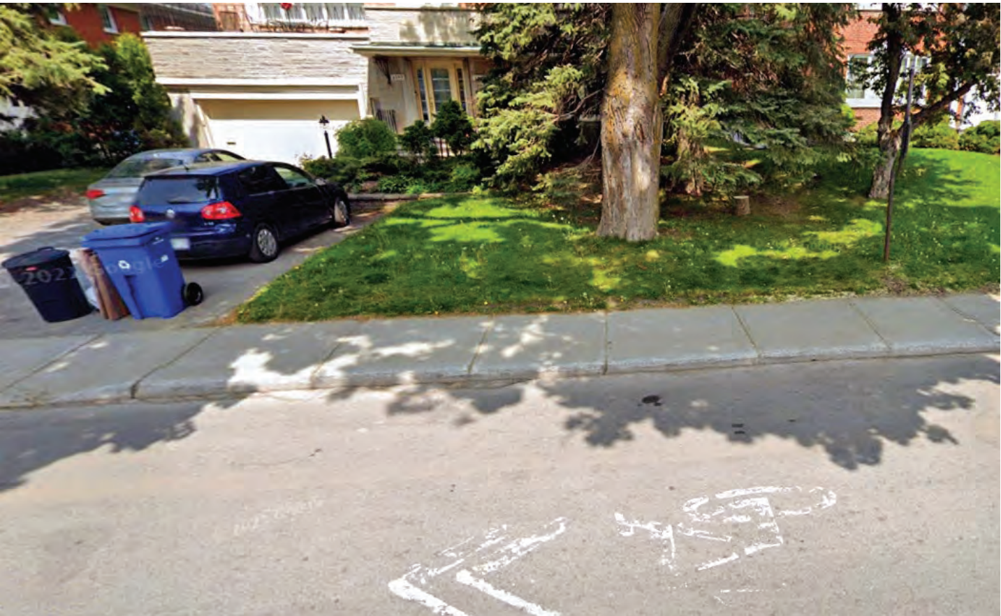
As seen here in this photo of the pavement along Graham Blvd., the faded outline of a designated bicycling route is apparent on the street surface, although it is not an officially-designated bicycle path.
