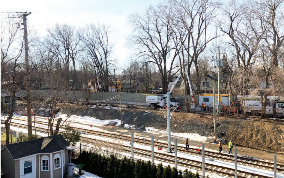
Photo: A view looking towards the western side of the REM train line last week of contracted tree management employees working beneath the canopy of century-old trees on the closed Canora Road pathway.
